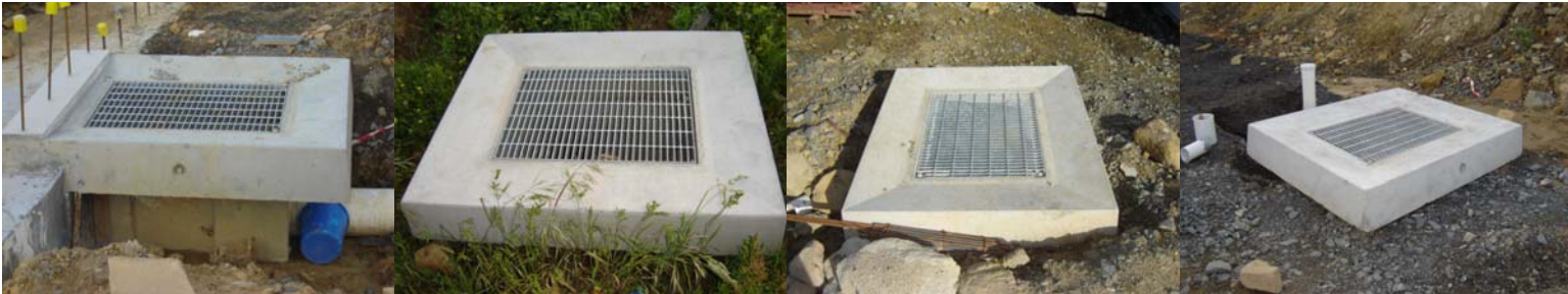
KSD 3-03 GRATED STORMWATER PIT
