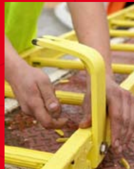
Bolting on the wall brackets
