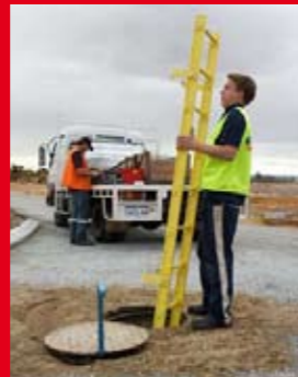
Ready to install the ladder
