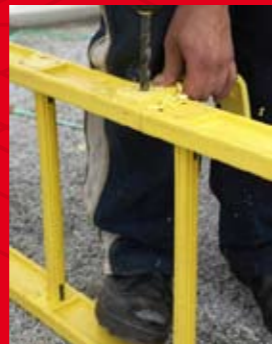
Drilling in the wall brackets
