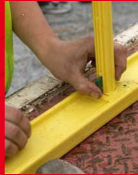
Placing in the retaining clips
