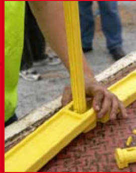
Assembling stile and rung
